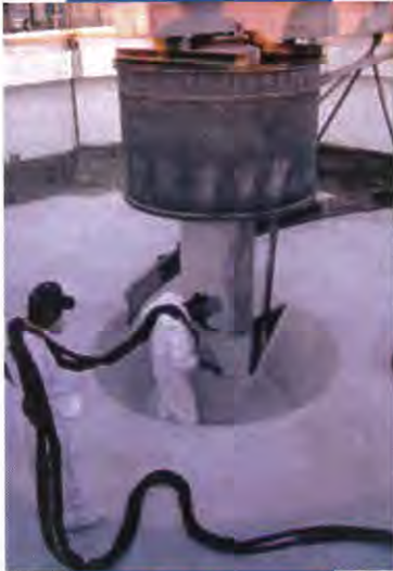
Particulars of a Purtop 1000 waterproof coating applied on various substrates (cementitious and metallic)
