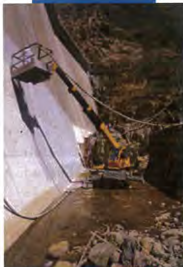
Waterproof coating on a dam
